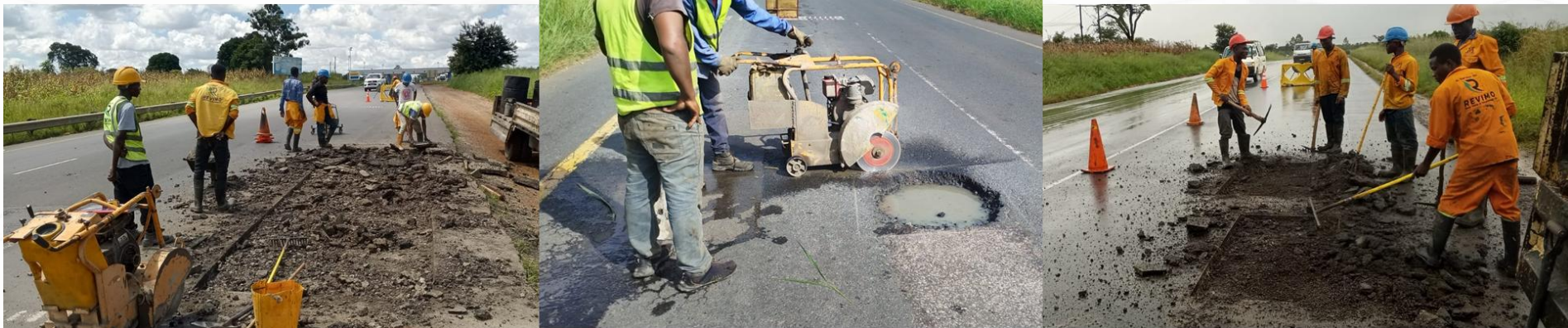
Figura 26 – Tapamentos de buracos nos troços Beira - Tica e Manica - Inchope / Figure 26 - Patching Potholes on the Beira Tica and Manica Inchope Roads
